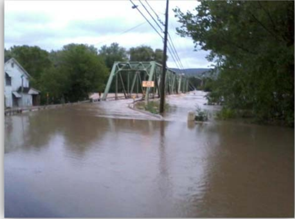
Figure 1: Bridge Street during the flood.
