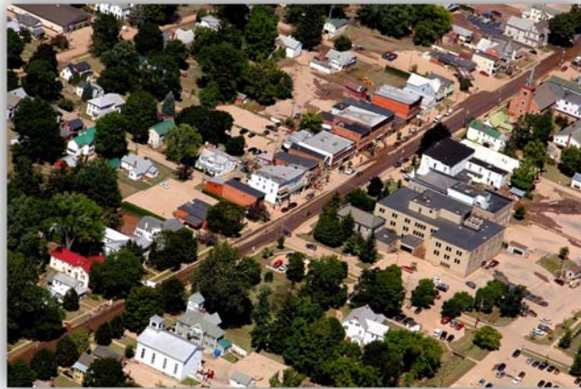
Figure 6: Aerial view during the flood.
