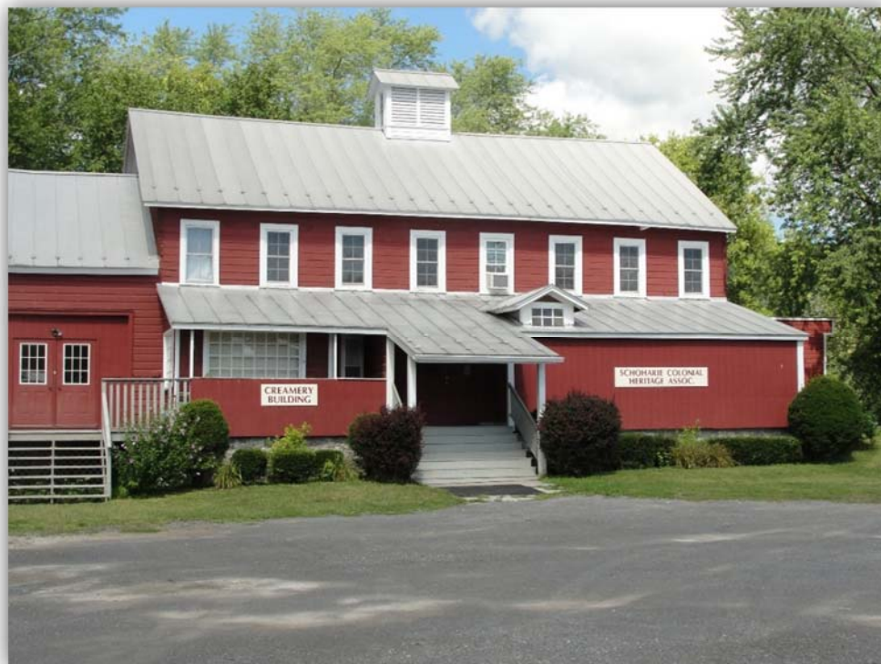
Figure 10: The Creamery Building, Schoharie Colonial Heritage Association on Depot Lane.
